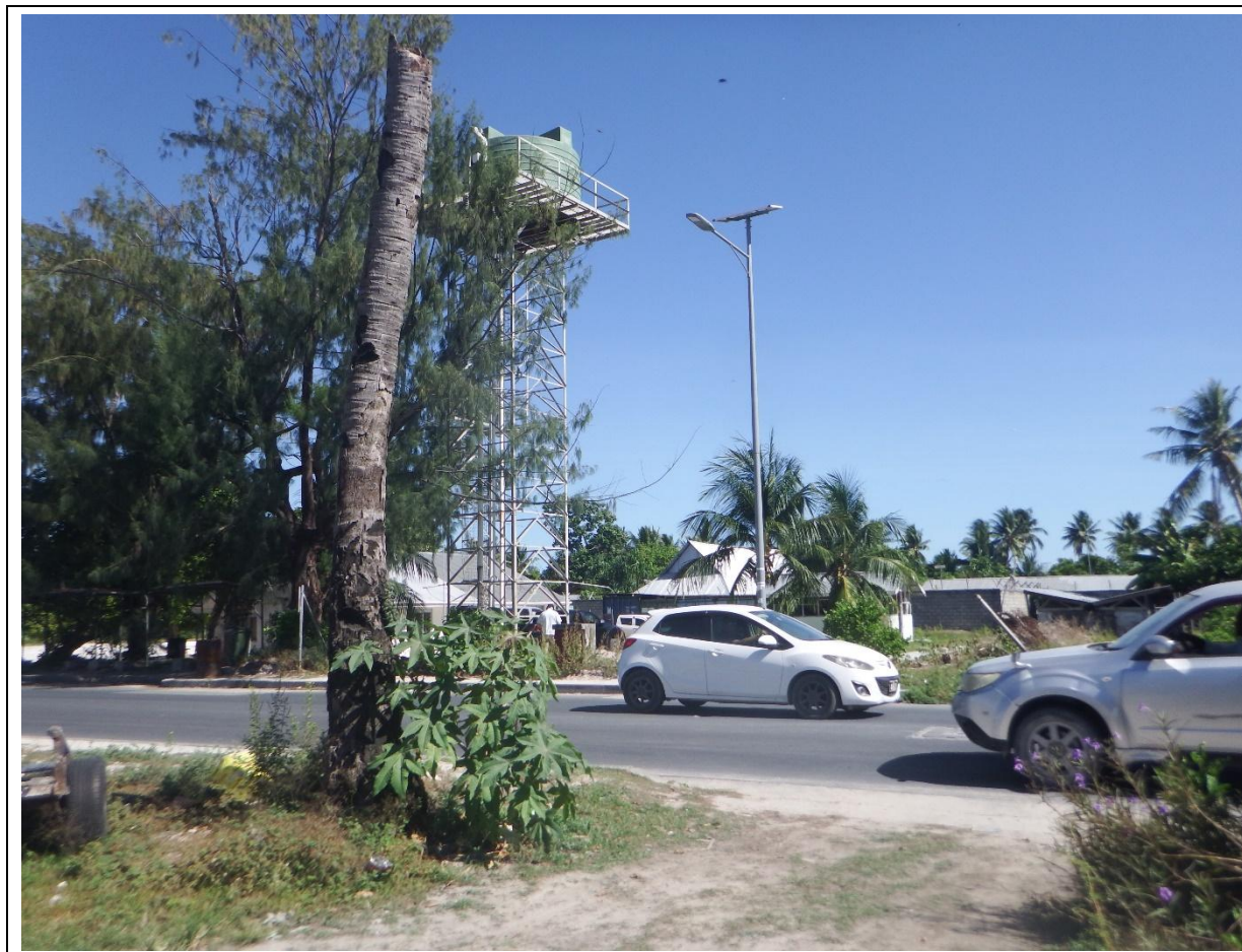
Figure 8: Salt Water Elevated tank on Tower Betio
